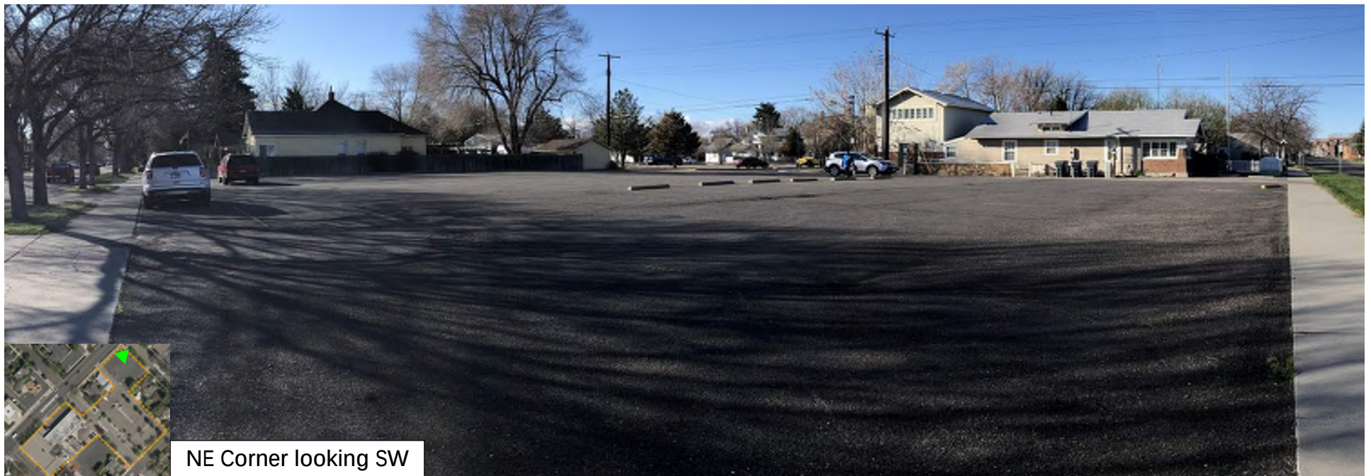
Rear Circle Drive Area
