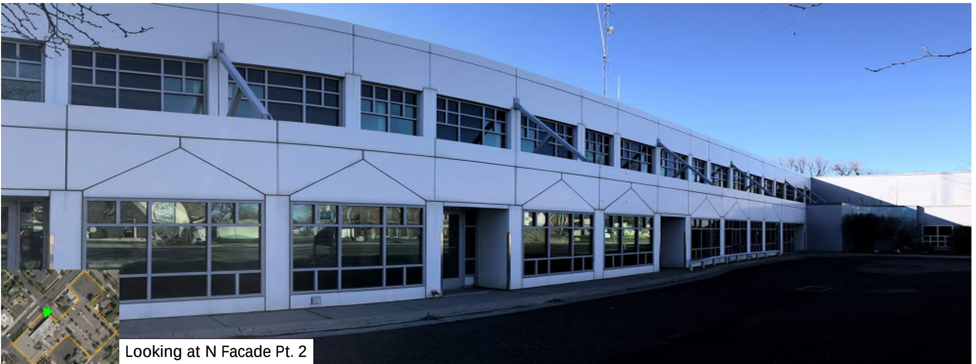
Looking at N Facade
