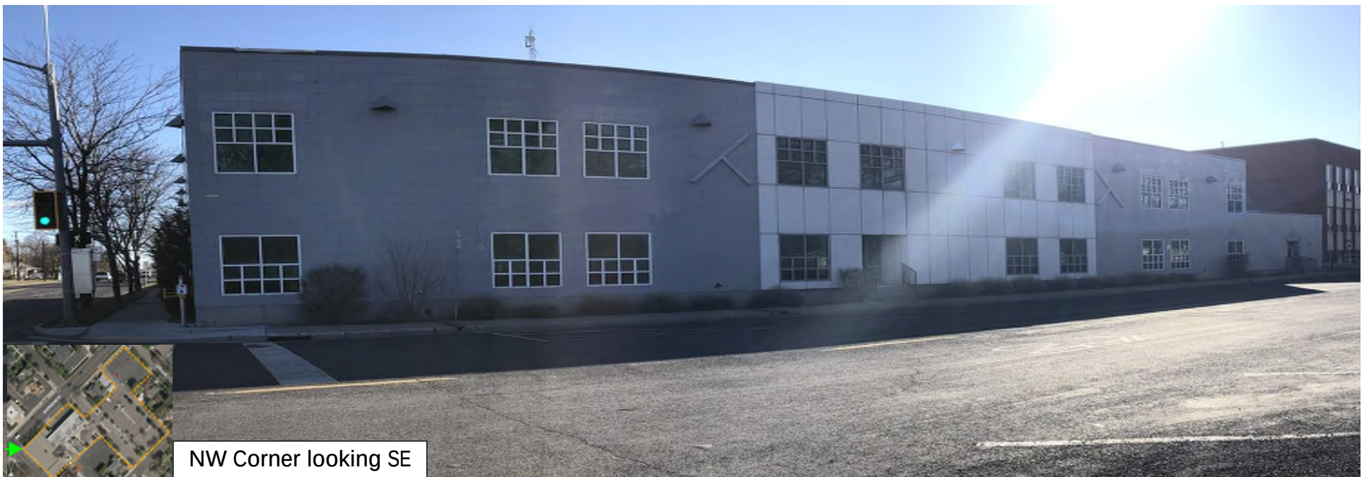
SW Corner looking NE
