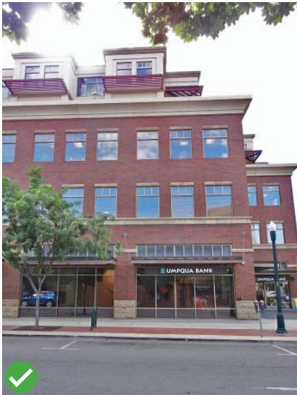
Proportion relates to surrounding buildings.
