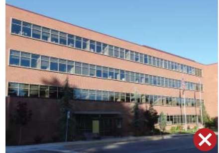
Inappropriate openings on facade.
