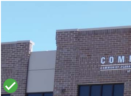
Acceptable parapet detail.
