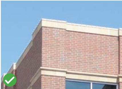
Acceptable parapet detail.
