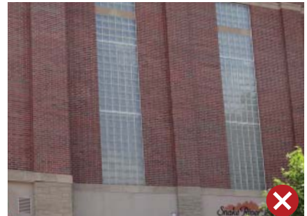
Inappropriate scale and proportion of opening.
