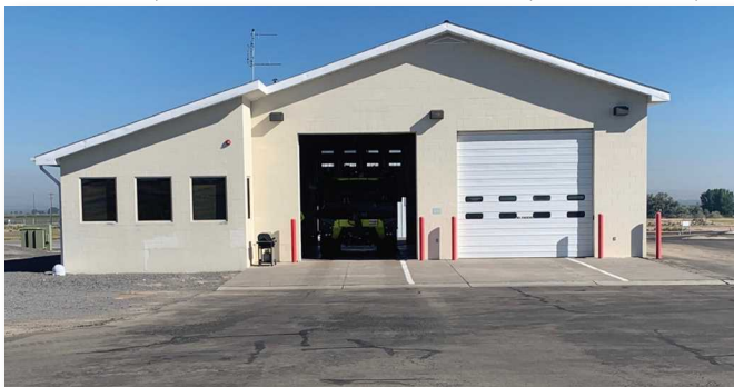
Joslin Field, Magic Valley Regional Airport > Architectural/Engineering Service
