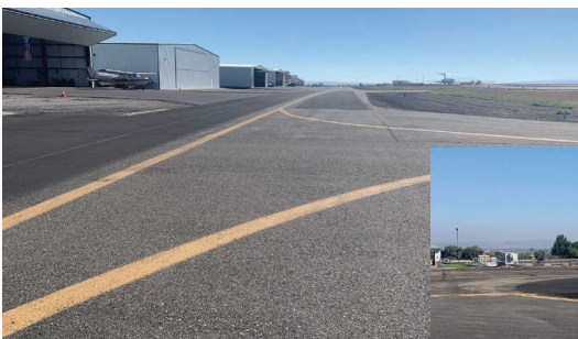
Taxiway L Construction
