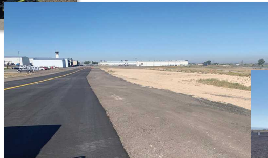
Taxilane 14 Extension and Cargo Apron Construction
