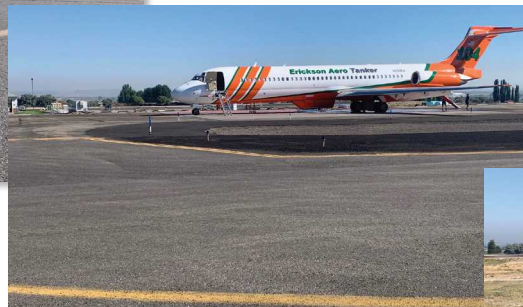
Taxiway A Reconstruction and Realignment
