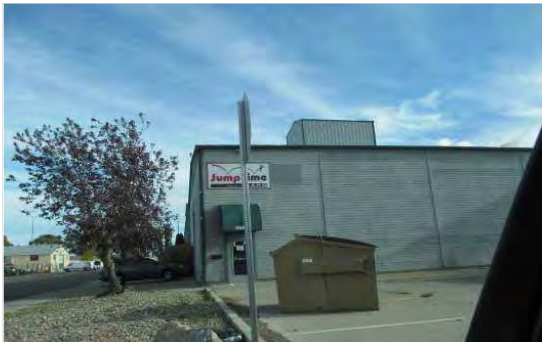
3 rd Avenue South & Idaho Street
