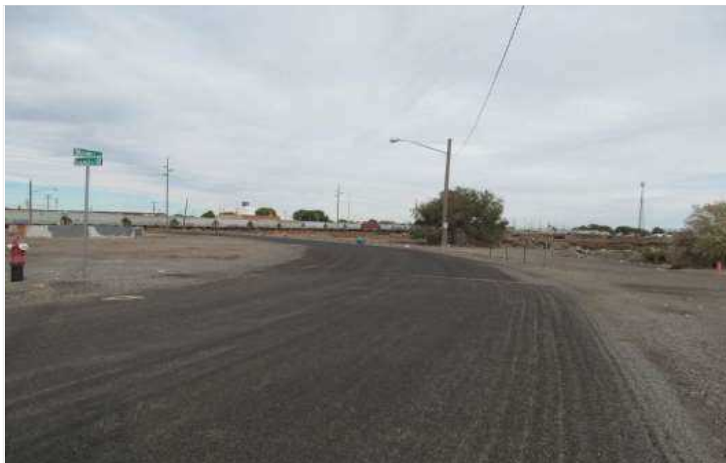
Looking East on Maxwell Avenue
