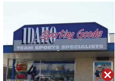
Inappropriate plastic, backlit sign.
