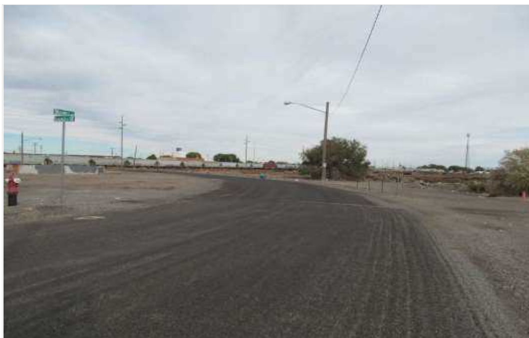
Looking East on Maxwell Avenue
