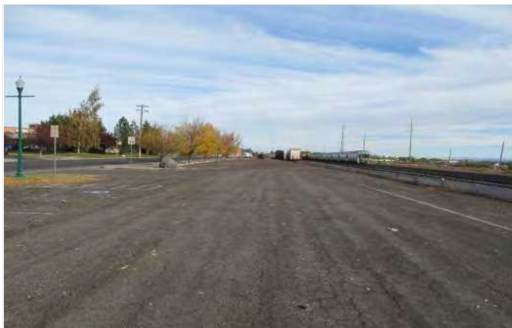
South Side of Minidoka Avenue & Hansen Street
