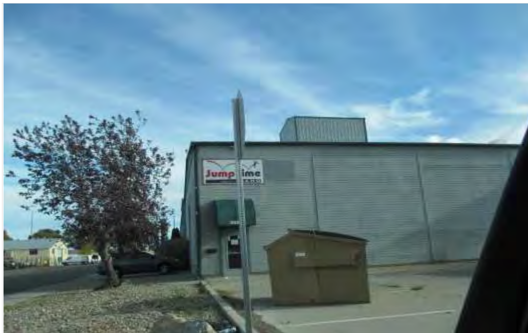
3 rd Avenue South & Idaho Street
