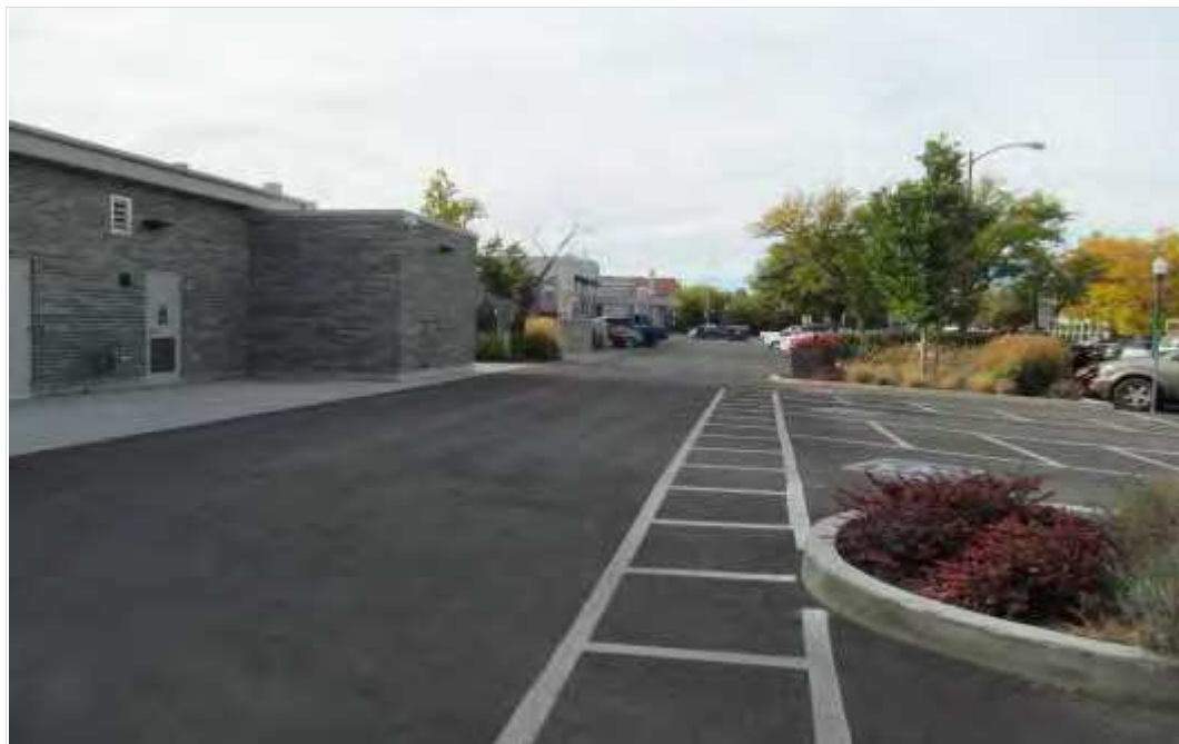
Paved Alleyway Looking North
