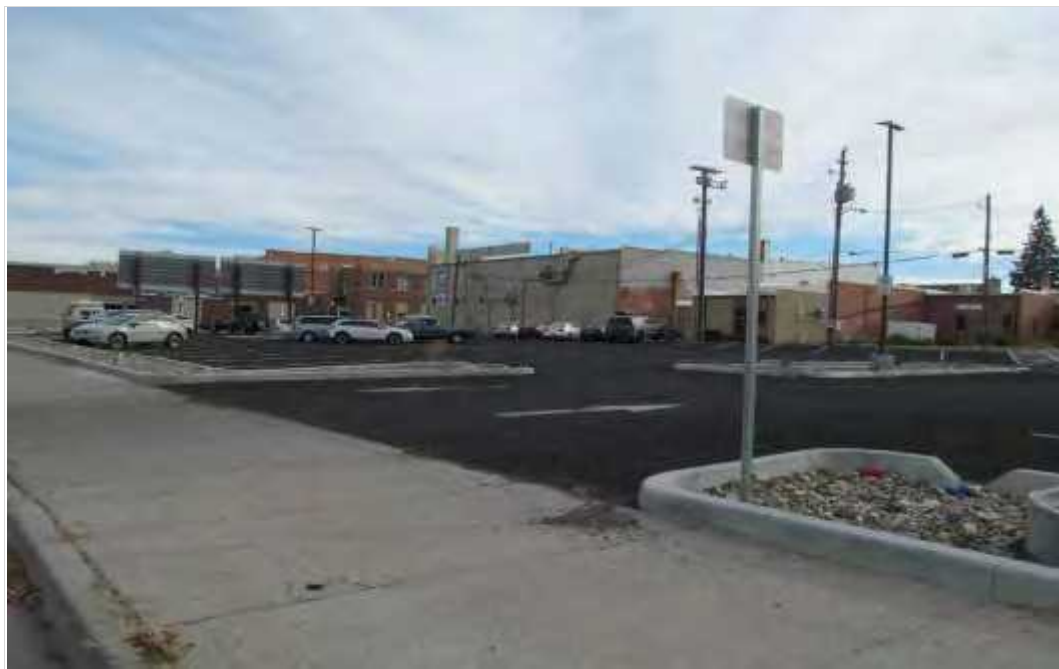
241 2 nd Avenue East Looking South
