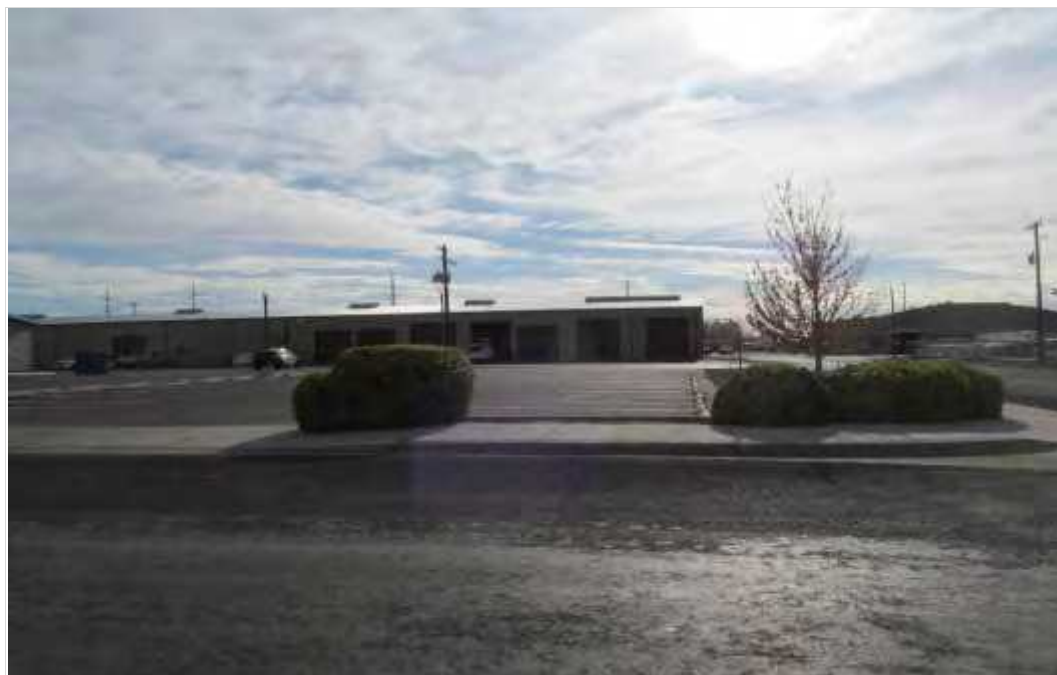
5 th Avenue West & Gooding Street Looking South West
