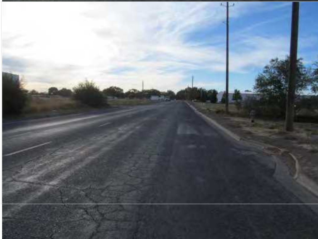
Victory Road Looking West
