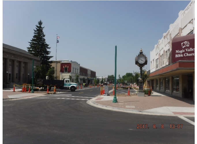
Block 2 – Gooding to Fairfield, block is open to traffic and installing landscaping, 08AUG2017
