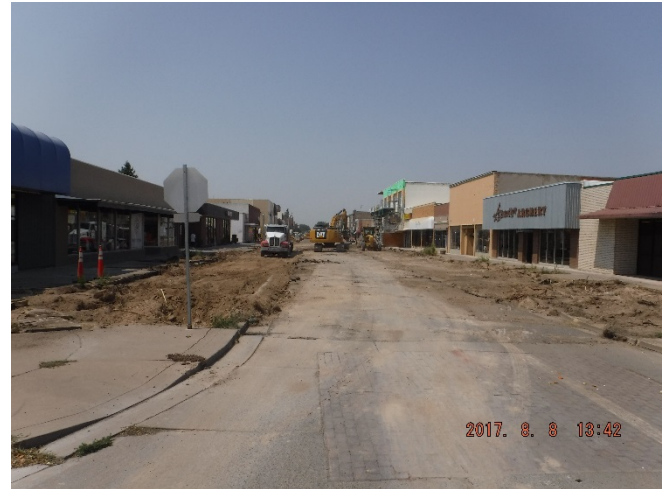
Block 4 – Hansen to Idaho, asphalt pavement demolition, 08AUG2017
