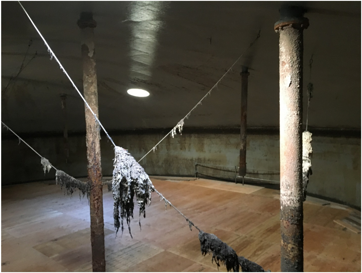
Photo 1: Overall view of digester interior
