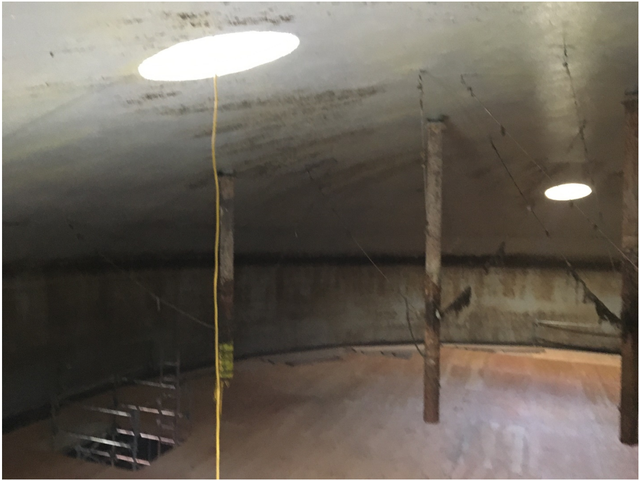
Photo 2: Overall view of digester interior
