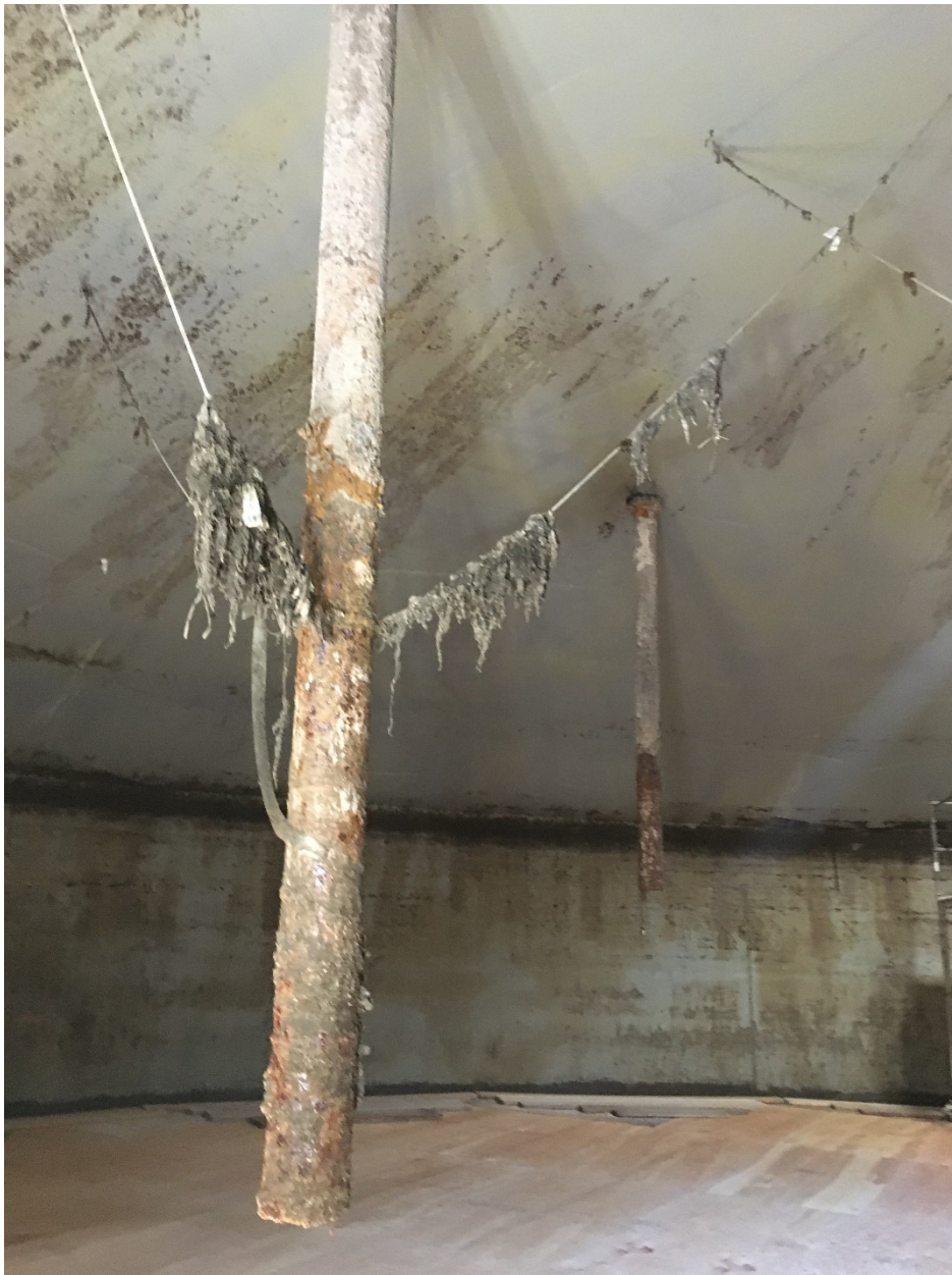
Photo 4: Sampling wells and overall view of digester interior
