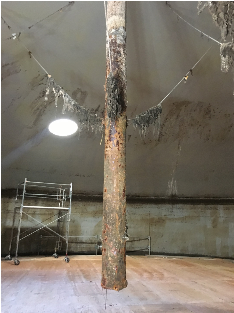
Photo 3: Sampling well and overall view of digester interior
