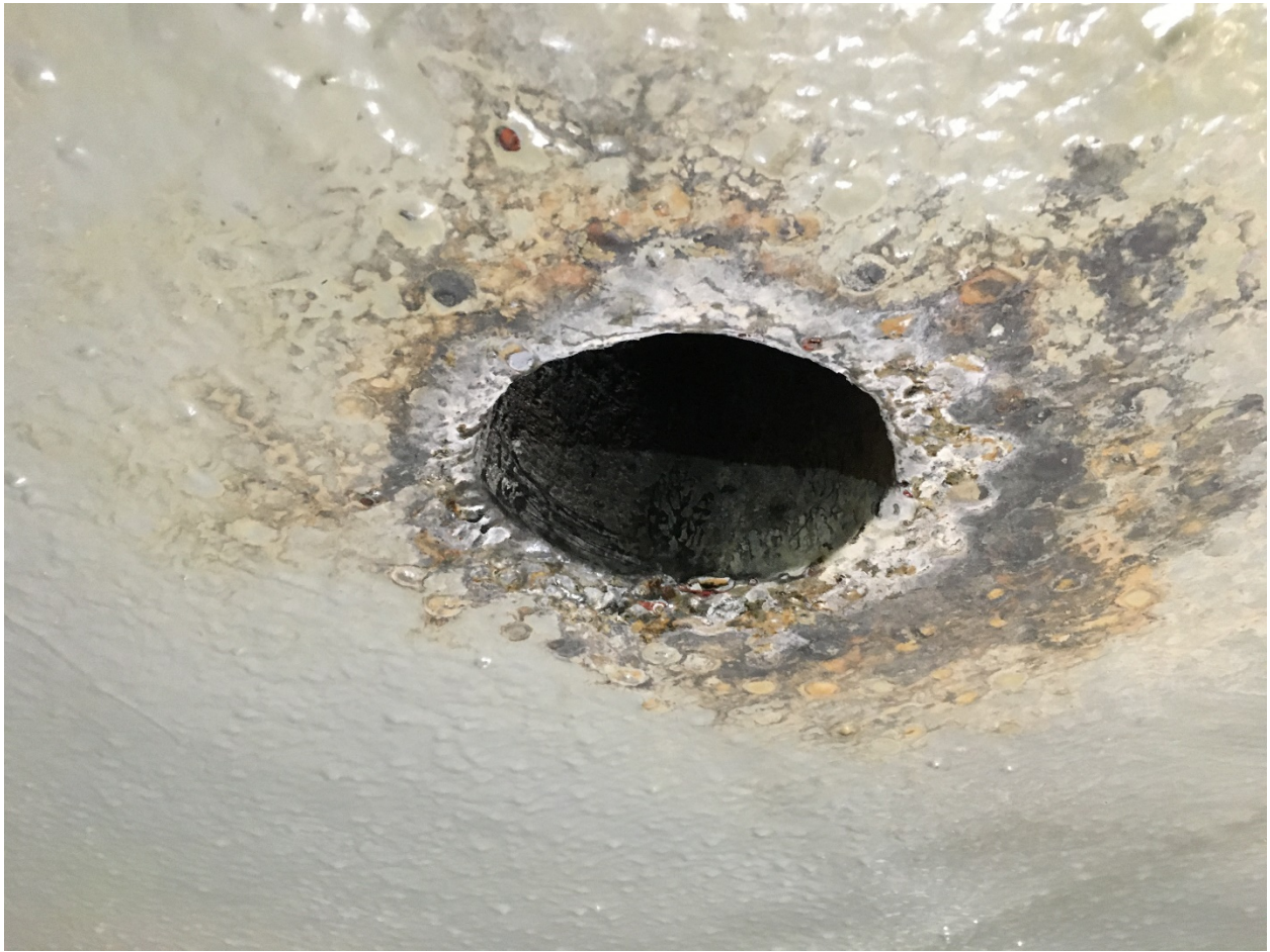
Photo 7: Flush port on the digester cover interior showing well adhered coating
