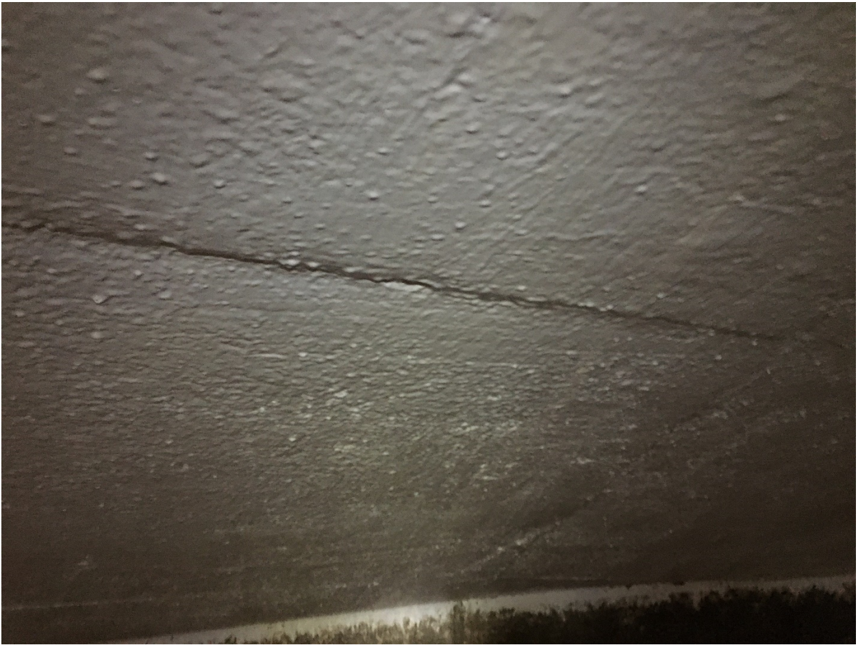
Photo 6: View of digester cover interior and form joints, both showing well adhered coating
