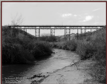
The Twin Falls train depot can be seen just east of the bridge. In March 1916, the city condemned the Shoshone Street Bridge. It was replaced in 1920 by what later became known as the Singing Bridge. The Singing Bridge, which hummed when cars drove over it, was replaced by the Old Towne Bridge in 1992.
