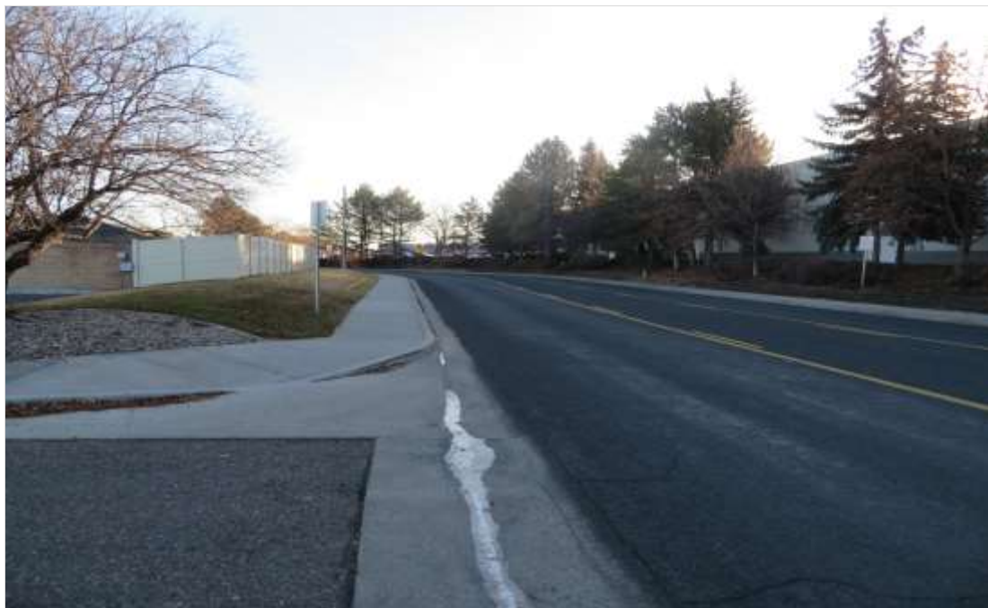
Fillmore Street looking east
